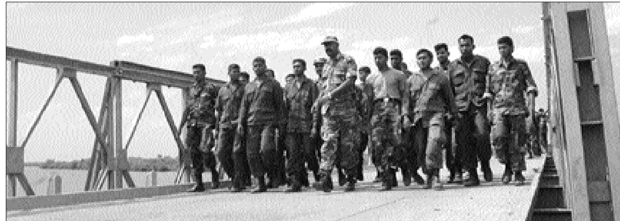
The Panichchankerni bridge repaired by the engineering troops.
