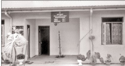
The new Samurdhi and Agricultural Research office building at Sagaragama, Nattandiya which was opened by Skills Development Minister Dayashritha Tissera recently. (Picture by Puttaram District Roving Corr.)
